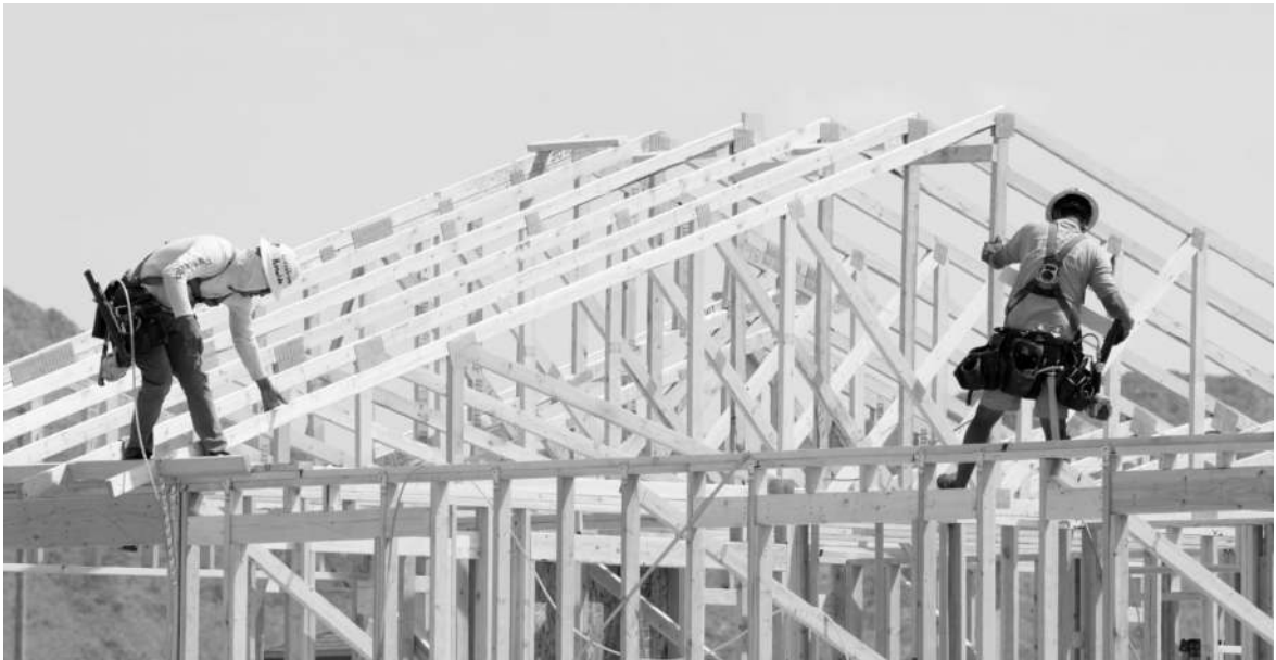
Ross D. Franklin/AP Construction workers frame up a roof of wood lumber at a new home build, April 1, in Laveen, Ariz.
